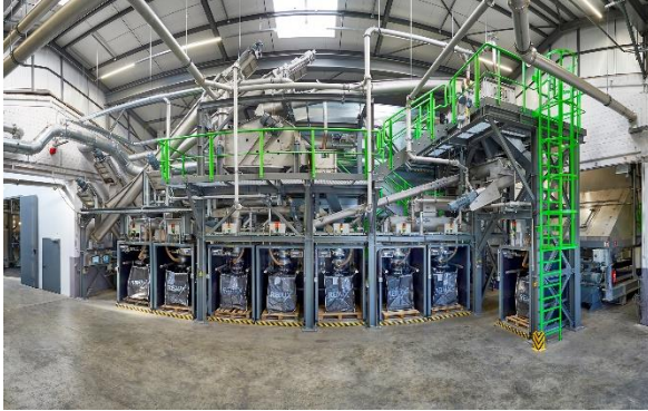
Photo 1: R: Recycling plan for all types of lithium batteries in Bremerhaven. Photograph rights: Saubermacher.
